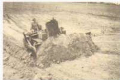
Howard building dam.
