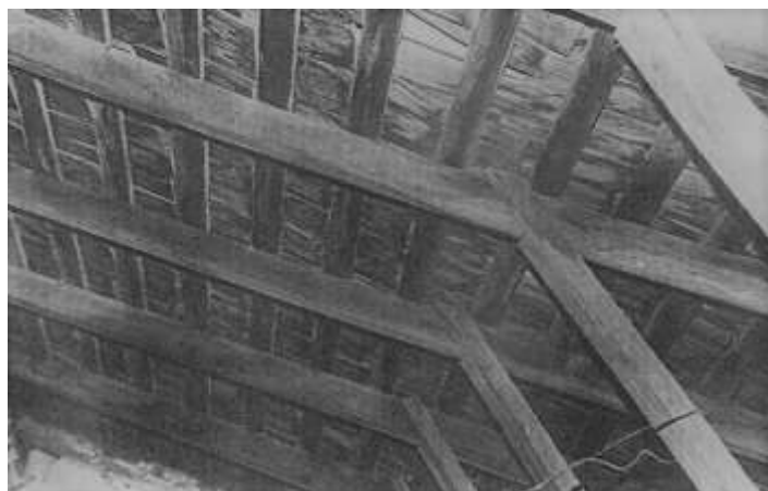
Shingle roof on Drury's coolroom, now covered with iron
